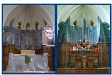
Pedal pipes, except for the largest wooden basses, covered their windchests with plastic sheet and plywood, closed and sealed the Swell and Choir expression shutters, and built a
