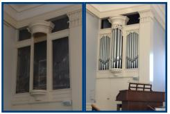
In April 2018, we removed the façade pipes and pipe shades from the twin cases of the 55 rank Roche organ, Opus 34, sealed off both organ chambers with plastic sheets, and
